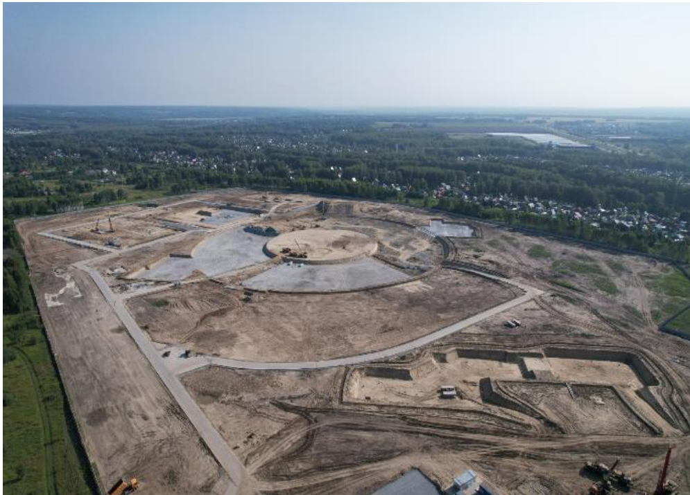
Fig.1. Construction site of the Synchrotron Radiation Facility SKIF (as of summer 2022).
